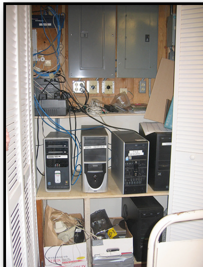
The famed "back room" server closet at the John C. Fremont Library (CO), MaintainIT, http://tinyurl.com/dhc6za
